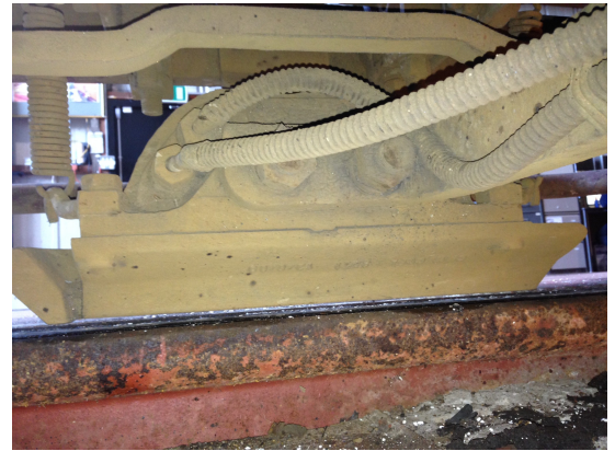
392's track brake. Photo taken from in the inspection pit
